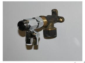
This photo shows the braided line adapter fitted. All that is required is to unscrew the braided line off the mains supply and install the adapter. The supplied black washer is to be installed into the female thread end of the adapter .Once the supplied adaptor is fitted, you can re-install the braided hose to the  $\frac{1}{2}$ " male thread.
