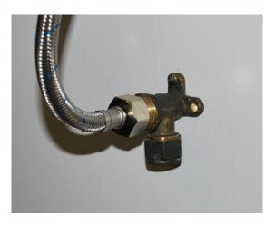
This is a braided line and normally used to connect a flick mixer type tap to the mains supply. Braided hoses are normally fitted finger tight, if you do use multi-grips to tighten, do so gently as excess pressure is not required. Remember to turn off the water supply.
