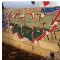
Filled-in bubble writing on previously coated masonry wall.
