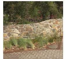
Once clean, re-apply WBGC.
