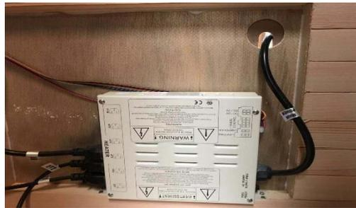
B. Connect and screw the 'CTRL' connectors together to provide power to the control panel.
