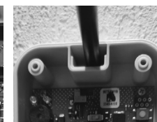
Fig. 10: Marking the drill holes
