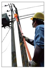
Check and detect live high voltage cables(using extension hot stick.)
