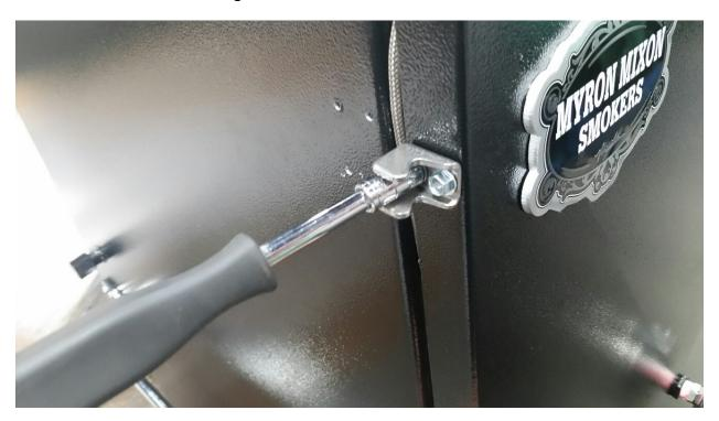
6. Install new Clamp and Tighten screws.
