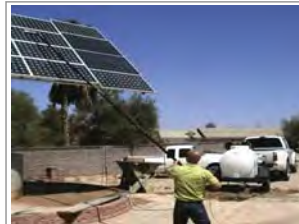
SOLAR PANEL CLEANING
