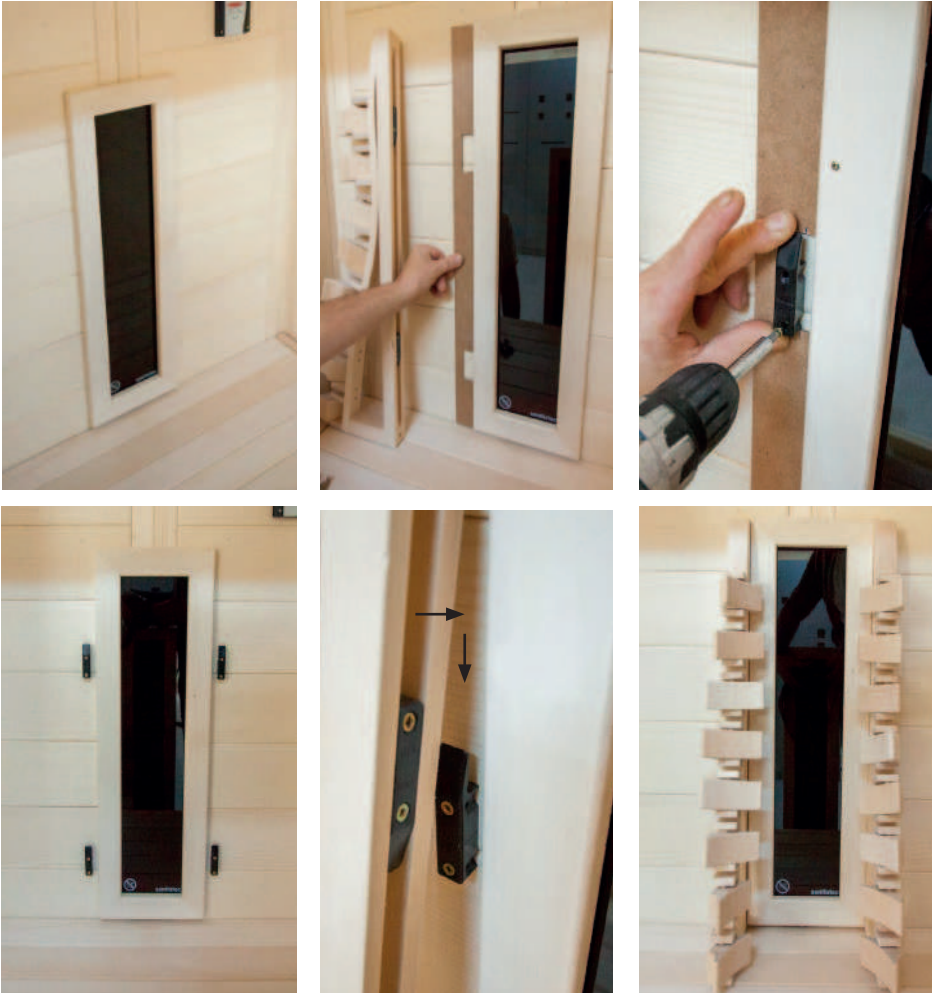
Fig. 29: Installing the backrests
