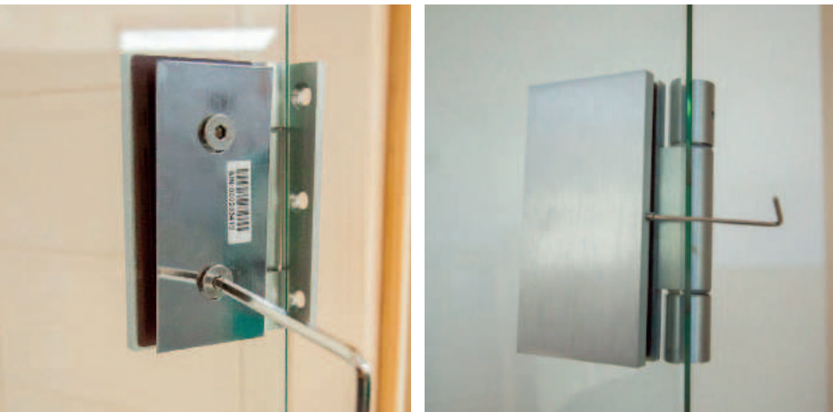
Fig. 32: Installing door fittings 2
