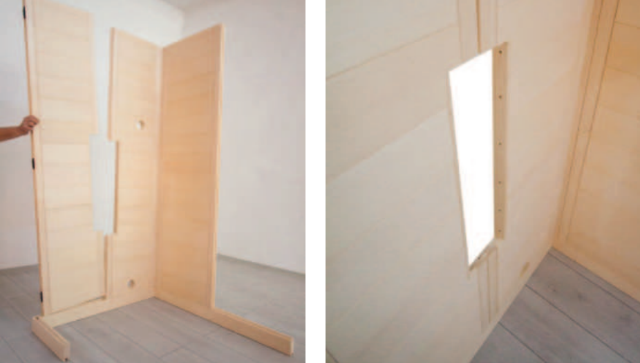
Fig. 6: Inserting wall element with recess
