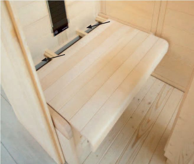
Fig. 28: Attaching the bench
