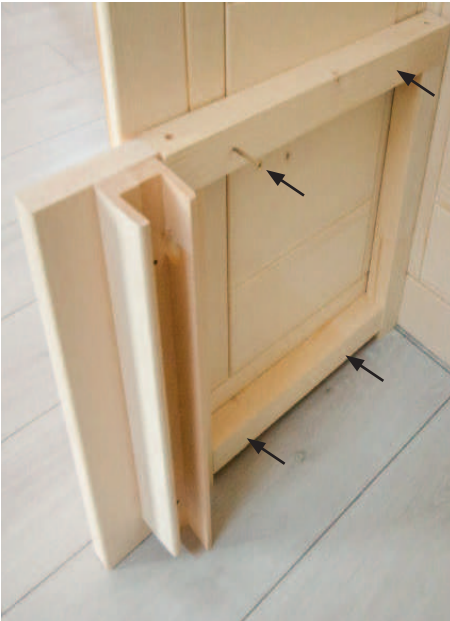
Fig. 18: Installing the bench supports
