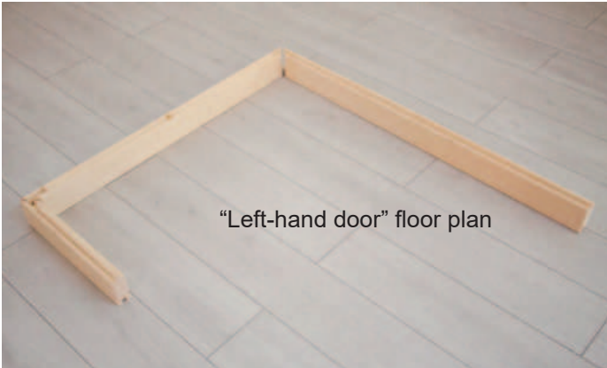
Fig. 1: Laying the three base frame elements
