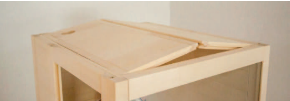
Fig. 15: Fastening the ceiling elements
