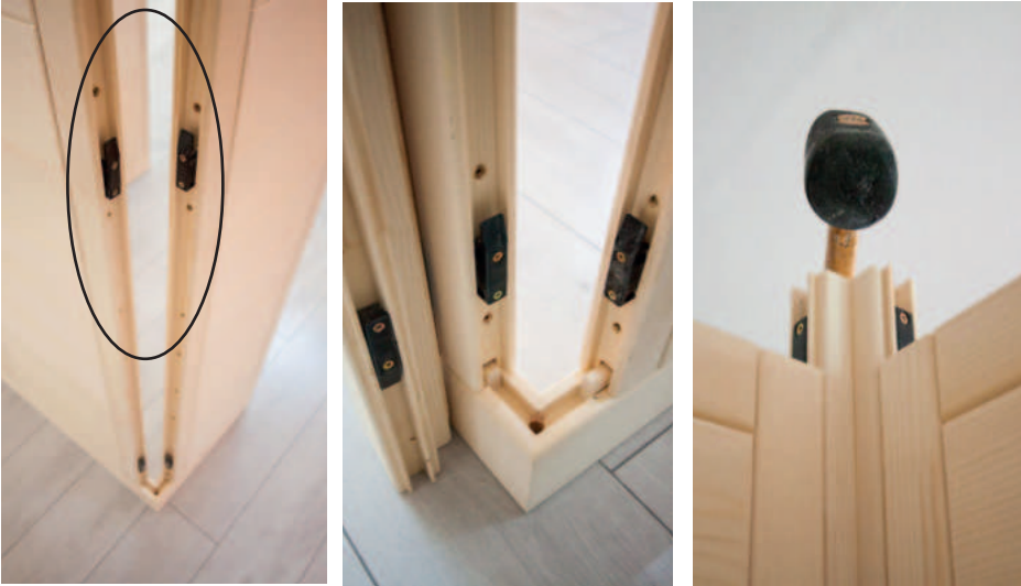
Fig. 4: Connecting wall elements with corner post
