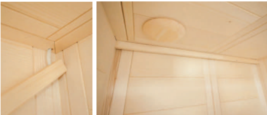
Fig. 24: Attaching the LED strip
