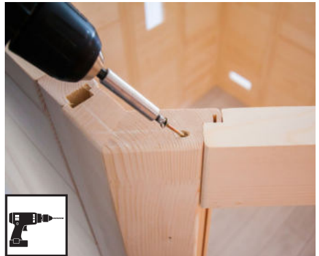
Foret de 3 mm, 1 vis 4 x 70 mm
