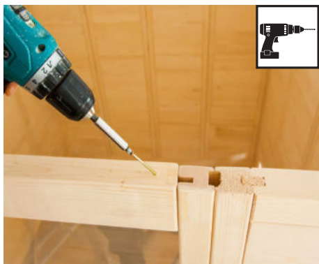
Foret de 3 mm, 1 vis 4 x 70 mm
