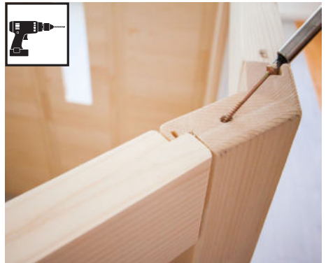
Foret de 3 mm, 1 vis 4 x 70 mm
