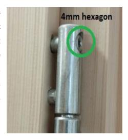
Fig.2 Frame horizontal direction adjustment bolt
