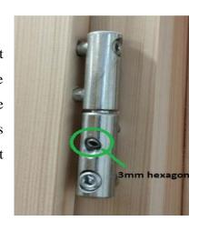
Fig.1 Sash hinge height adjustment bolt
