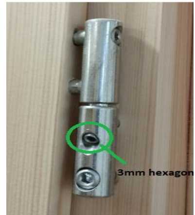
Fig.1 Sash hinge height adjustment bolt
