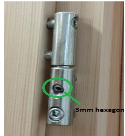
Fig.1 Sash hinge height adjustment bolt
