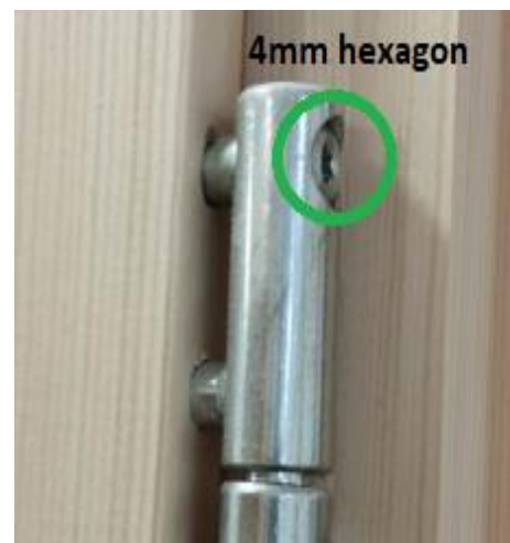
Fig.2 Frame horizontal direction adjustment bolt
