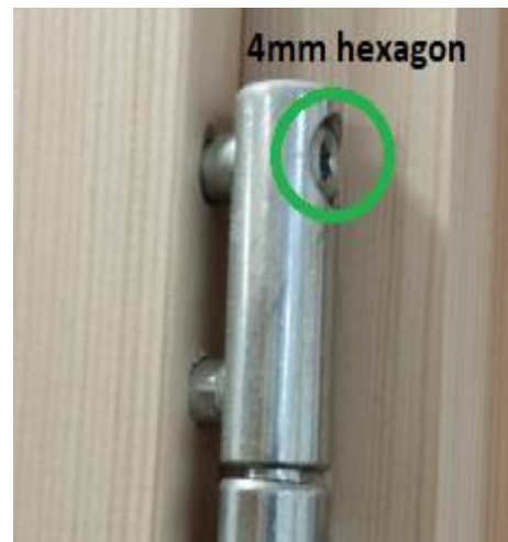
Fig.2 Frame horizontal direction adjustment bolt
