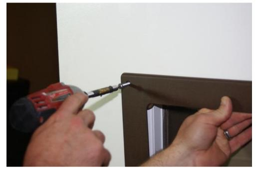
11) LEVEL THE DOOR AND REPEAT STEP #8, #9, & #10 MARK, DRILL & TEMPORARILY INSTALL UPPER CORNERS WITH TAMPER RESISTANT SCREWS. NOW MARK BOTH BOTTOM HOLES, REMOVE DOOR, AND DRILL THE BOTTOM TWO HOLES. YOU ARE NOW READY TO INSTALL THE FRAME. FIRMLY TIGHTEN THE SCREW HARDWARE (APPLY THREAD-LOCK ADHESIVE) TO COMPLETE THE INSTALLATION.
