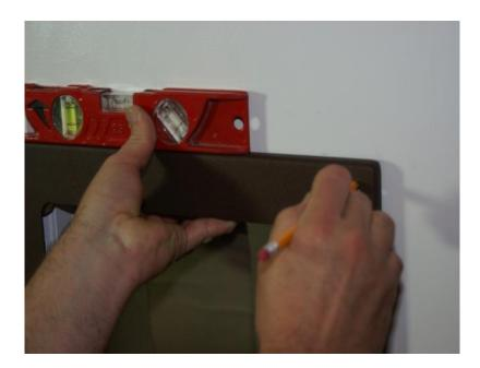
6) SET THE NEW SECURITY PET DOOR ON TOP OF THE EXISTING PET DOOR & MAKE SURE THE CENTERLINES ON THE VERTICAL SURFACE OR ON TOP OF THE FRAME LINE UP MAKE TWO MARKS ON THE SIDE ONE AT TOP AND ONE IN THE MIDDLE. YOU WILL USE THESE TWO MARKS TO CENTER THE DOOR LATER.
