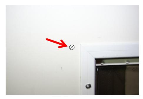
9) REMOVE THE DOOR AND DRILL THE CORRECT SIZE HOLE WHERE MARKED. THE SIZE OF THE HOLE WILL CHANGE BASED ON APPLICATION OF FASTENERS.
