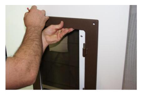
8) NOW USING THE TWO MARKS YOU HAVE MADE ON THE TOP, SIDES & CENTER TO SQUARE UP YOUR WATCHDOG SECURITY PET DOOR. PENCILE IN THE FIRST HOLE AT THE TOP CORNER OF YOUR WATCHDOG SECURITY PET DOOR. TO LOCATE THE POSITION OF FIRST MOUNTING HOLE TO BE DRILLED.
