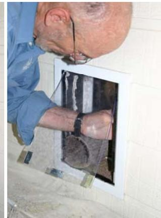
Apply the construction adhesive directly to the sides and bottom of tunnel.
