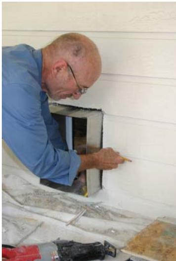
Hold pet door tightly against interior wall and mark with pencil from exterior to get correct tunnel depth.
