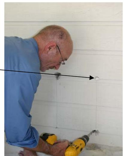
Drill out corners first to make it easy to insert saw blade.
