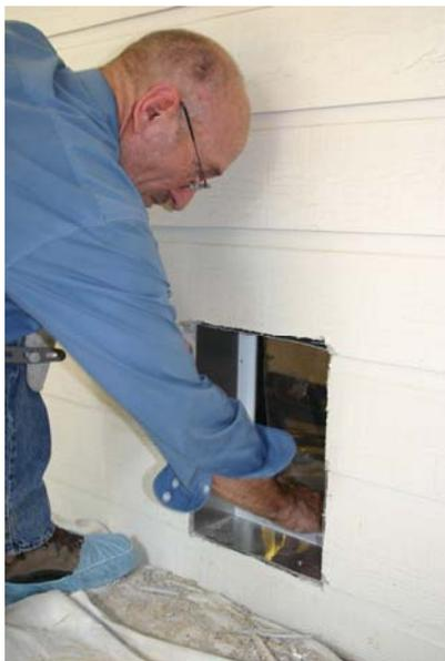
**Step 17:** Insert the inside frame and tunnel back into the opening. From the outside, pull the inside door frame tightly against the inside wall and push the flashing snug against the outside wall.
