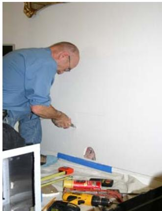
Cut the opening with a drywall saw.
