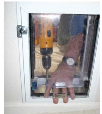
You should be drilling through one of your caulk beads when attaching the flashing to the tunnel.
