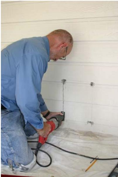
A reciprocating saw easily cuts the exterior hole, although other types of saw can be used.
