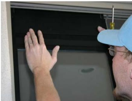
After loosening the adjusting screws, push the slide plates up until they stop and then retighten the adjusting screws with a Phillips head screwdriver.
