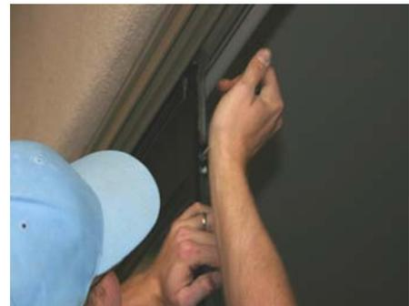
fuzzy weather-stripping between the edge of the panel and the edge of the adjustment unit. Cover it with a piece of foam tape (included).
