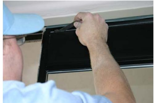
Use the wrench provided for the final tightening of the adjusting nuts
