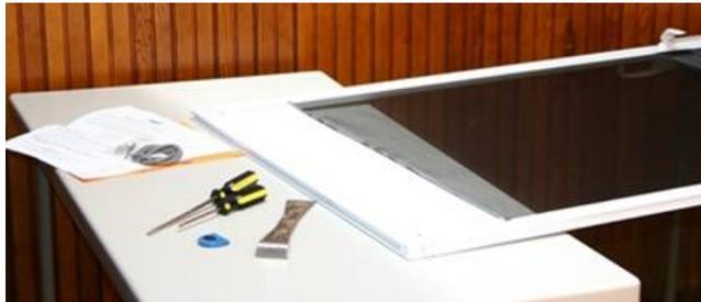
**Step 6:** Lay the screen window or screen door on a flat surface with the screen spline facing upward.
