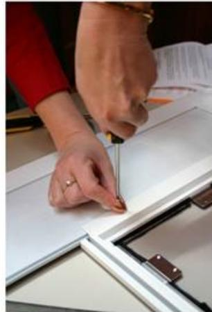
**Step 9:** Drill through the sides and bottom of the inner pet door frame and screen frame with the 7/64" drill provided. Insert the #6 screws with a Phillips screwdriver. Be sure the screws will not interfere with the operation of the screen door.
