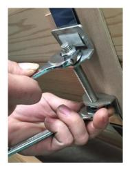
11.Install the benches inside barrel. Place the long benches onto the sides of the barrel using the supports at the front and back panels. In the center on the benchs underneath, install the 20cm 'Inside bench support beam' onto the side of the barrel wall using 2x '4\*40mm Screws'. Then screw the bench from the topside down into the support beams.
