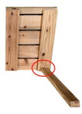
C. Place the bench seat and leg support onto the support beams. Secure the leg support into the barrel using 2x '4\*40mm Screws'
