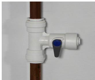
Identify a suitable length of 15mm mains cold water pipe work that is straight, clean and free from paint. Turn off the supply, drain down the pipe and remove sufficient pipe to allow for the pushfit tee to be fitted. The cuts to the tubing should be square and free from burrs. Ensure that the lever valve to the 1/4" branch is turned off before the water supply is turned back on.
