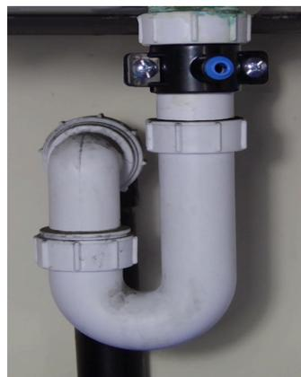
Push out the centre part of the self adhesive foam seal and remove the yellow backing paper. Stick the seal to the inside of the drain clamp, so it sits squarely over the hole.
