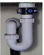
Push out the centre part of the self-adhesive foam seal and remove the yellow backing paper. Stick the seal to the inside of the drain clamp, so it sits squarely over the hole.
