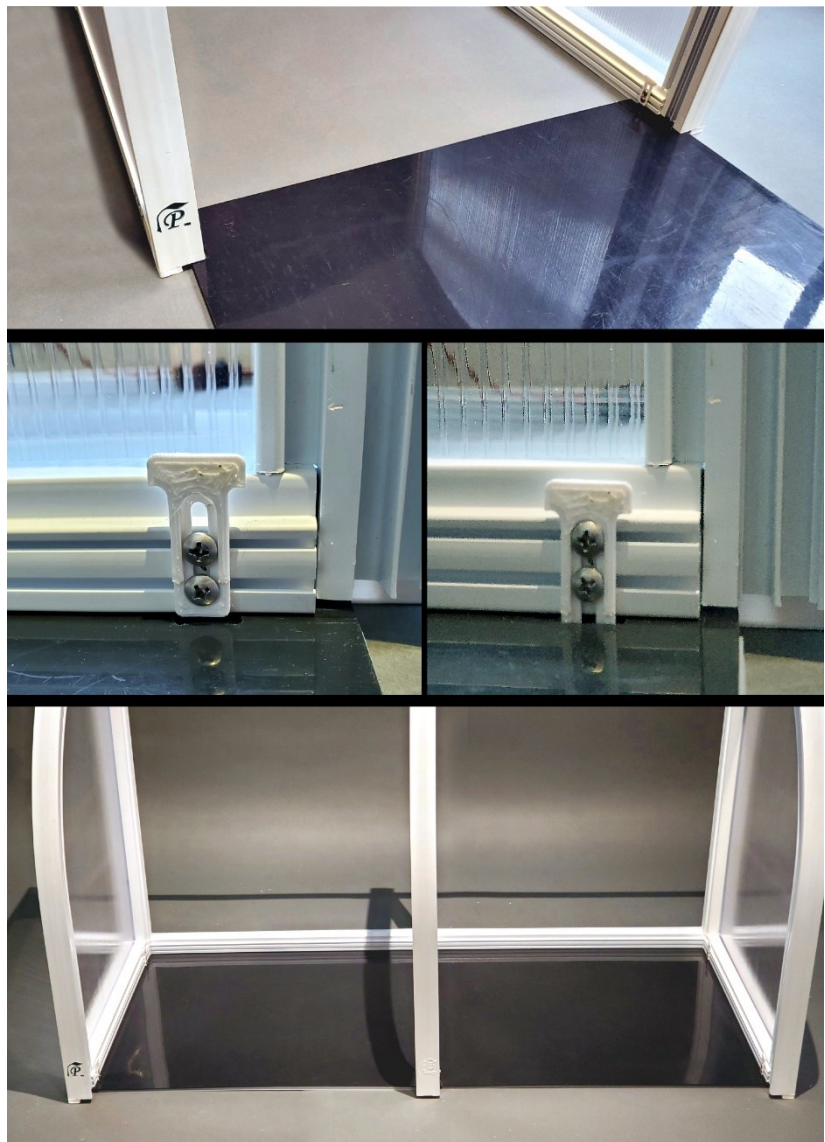
Figure 5 : Installation of the Base Plates
