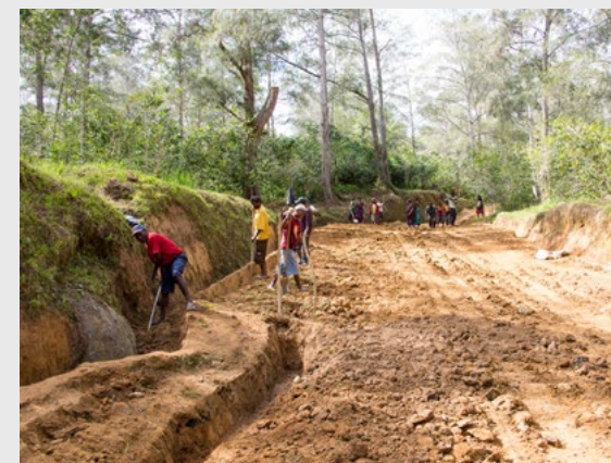
Road access improvements at HOAC, Eastern Highlands, PNG.
