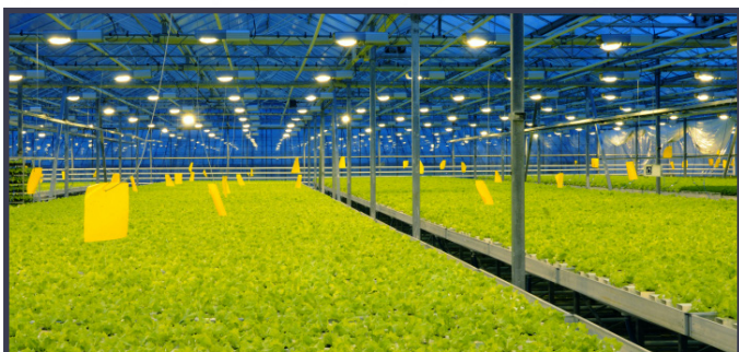
Greenhouse solar-supplementation using deep dish reflectors placed high above the plant canopy.
