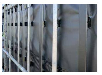
Tyvek® UV Façade Tape is a dedicated sealing tape suitable for sealing laps and bracket penetrations through Tyvek® UV Façade membrane
