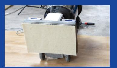
**2** Sanding with the **useit**® **Superpad P** grit 120 – when the old oil has been removed from the surface, the floor is then re-smoothed with a useit<sup>®</sup> Superpad P 100-150, following the recommendations of the oil manufacturer.
