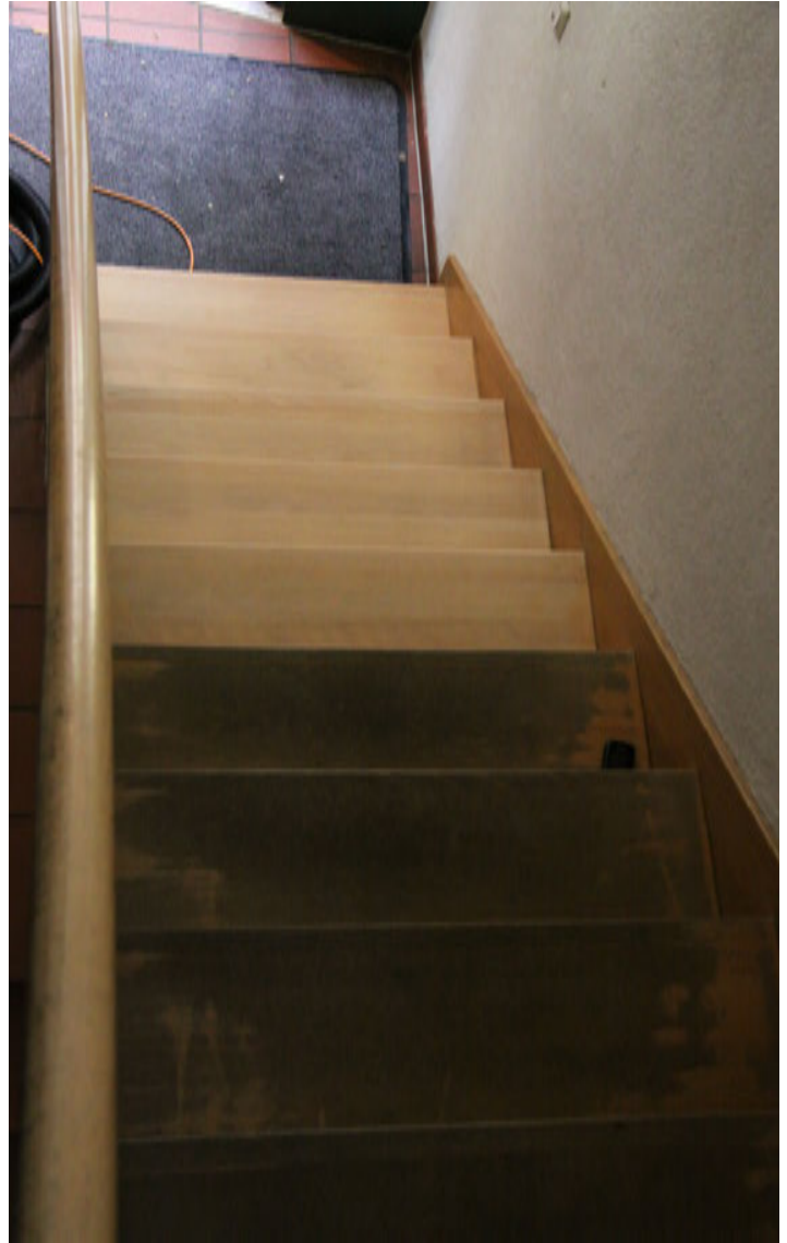
Sanding stairs with Jöst Big Boy orbital sander and useit®-Superpad P 40 yellow
