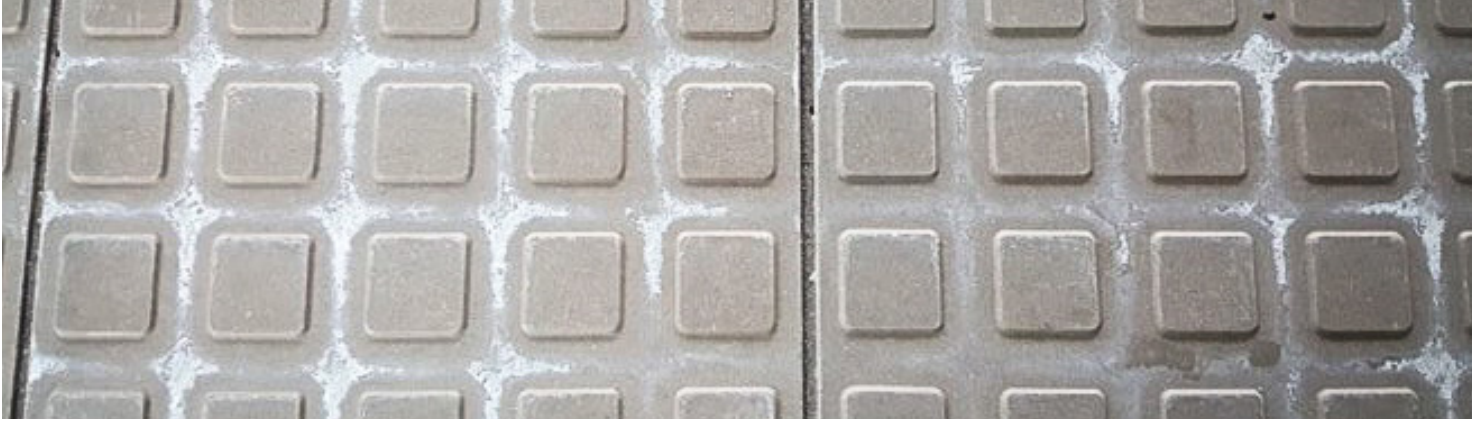
Removal of crystallization/calcifications with the special Abranopp® cleaning pad
