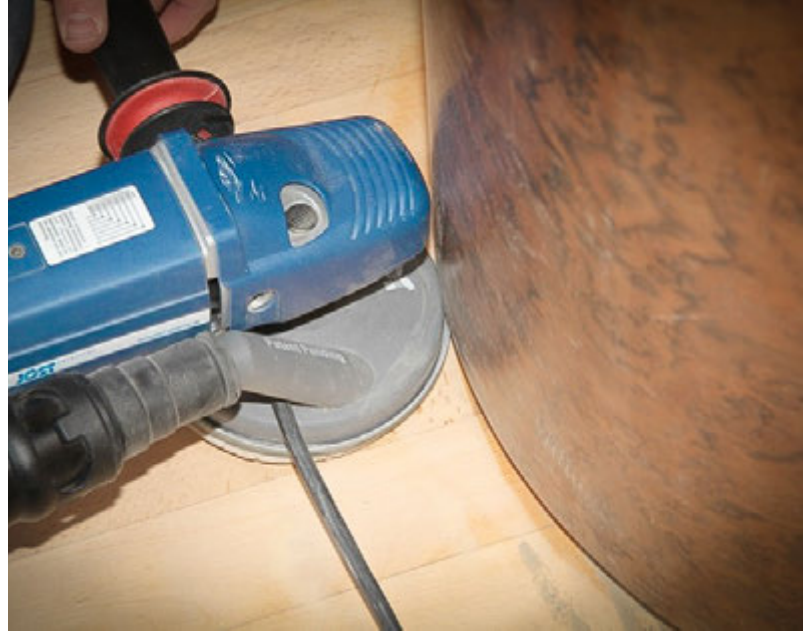
Straight-edged sanding with the P1 dust-free sanding system
