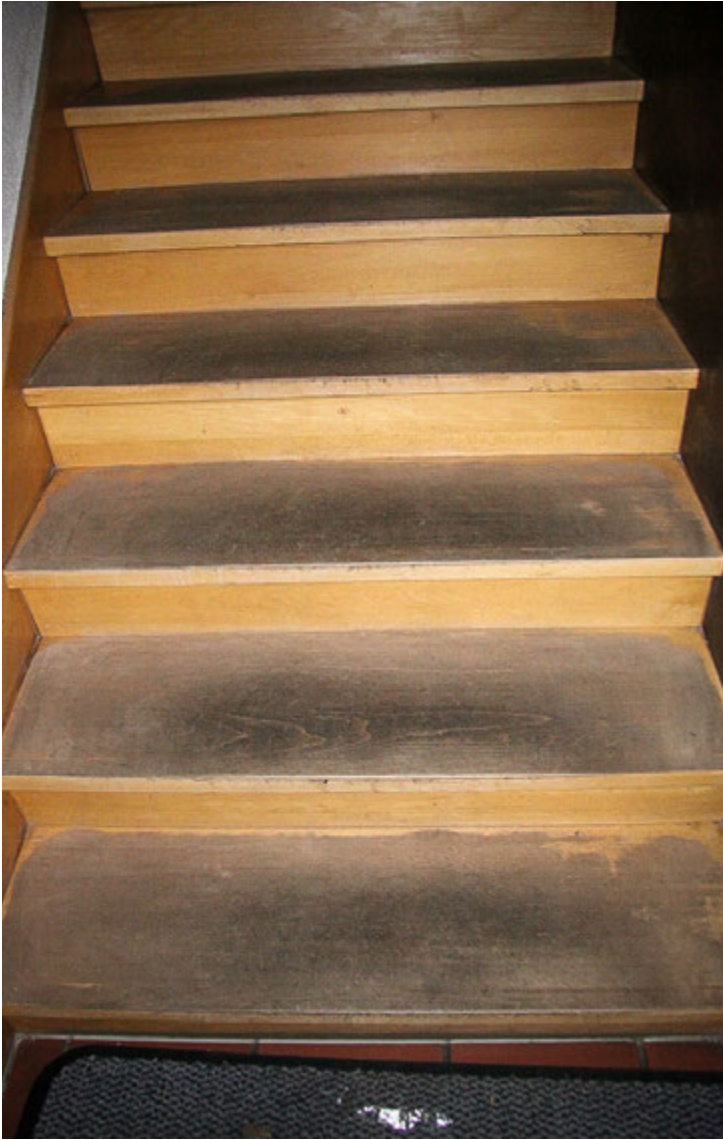
Sanding stairs with Jöst Big Boy orbital sander and useit®-Superpad P 40 yellow
