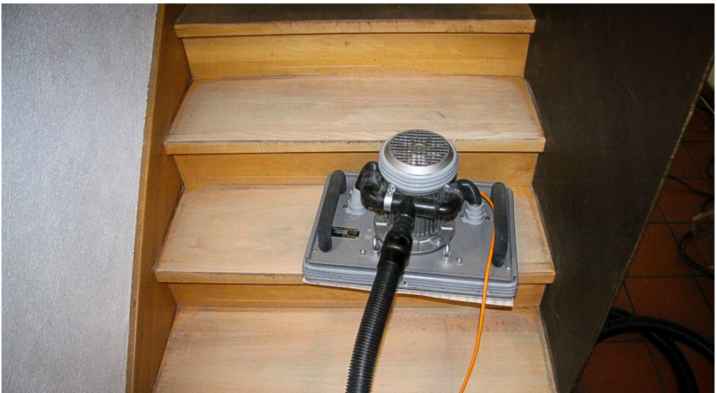
Sanding stairs with Jöst Big Boy orbital sander and useit®-Superpad P 40 yellow
