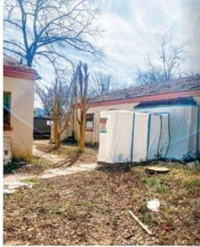
During the process of hazardous material remediation, the contractors place tarps over every door and window to make sure the toxic asbestos and lead particles stay inside the building and don't leak into the outside air. Even though the Villas are still in their decrepit state, locals and tourists alike drive by to see the activity and track the progress. "Everyone is excited, and that excitement is contagious," Sara says. "We can't wait to throw open the doors and welcome everyone in."
