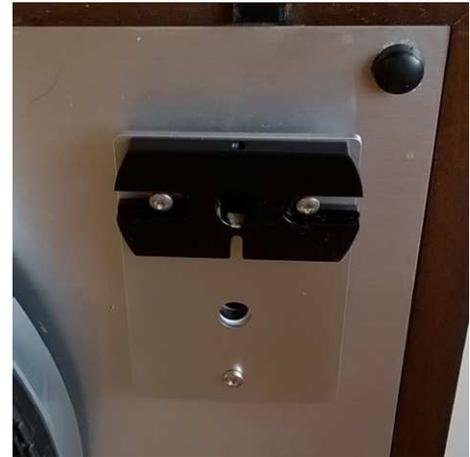
**Step 3;** Screw in but don't tighten. (Three screws)
