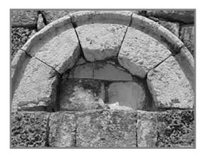
The arch above consists of five stones. The bottom stones on the left and the right are called "foundation stones." The middle wedged-shaped stone is called the "keystone."
