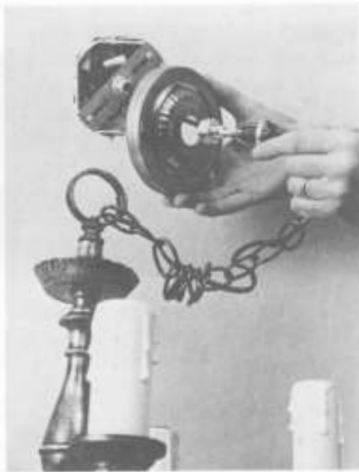
Attaching a chandelier to a square ceiling box
