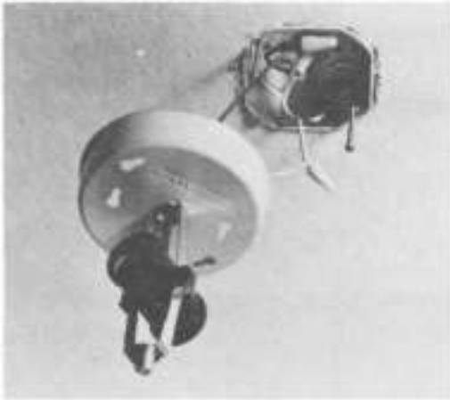
Canopy wired to ceiling outlet
