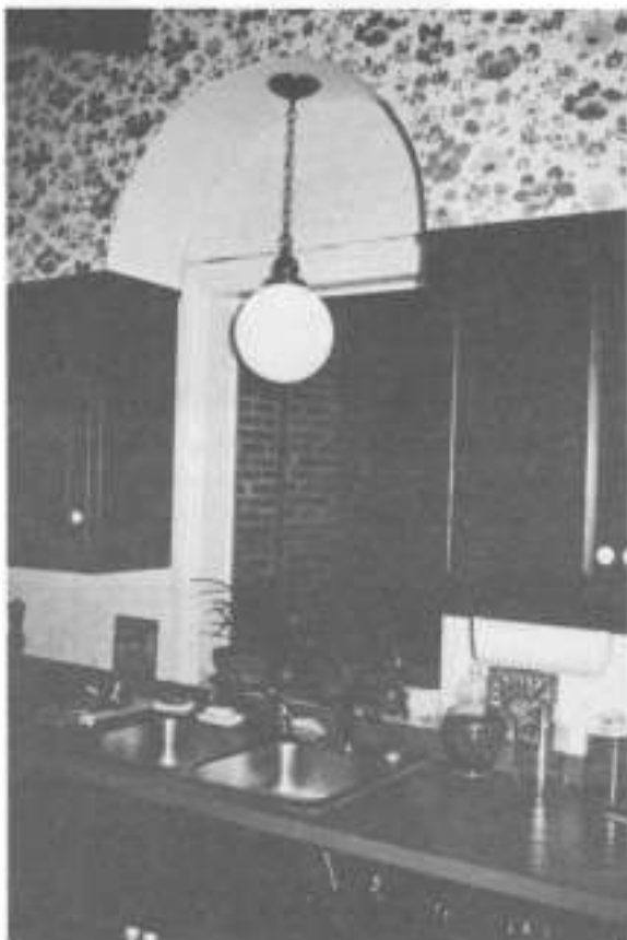
Ball of opal glass hangs by chain from an outlet over the kitchen sink. The globe opening has a neck that requires a shade holder with a 4" fitter.
