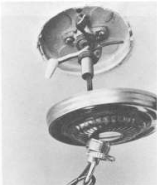
Attaching a chandelier to a stud-type ceiling box
