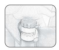
Pull up bottom circle connector Turn screw until tight Tension fabric with screws
