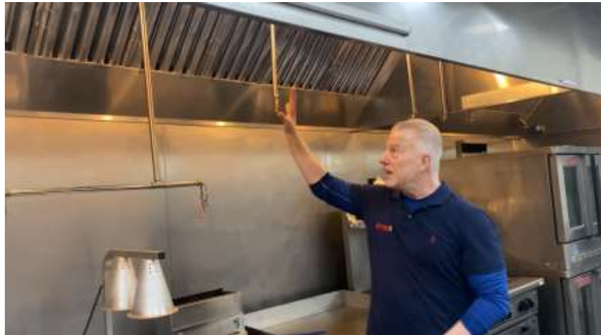
Figure 1 The kitchen's suppression hood, cleaned state
