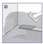
13. Comb out a layer of cement-based flexible tile adhesive to the limits of the waterproof membrane as drawn, filling any voids and maintaining the slope between the Sloping Board and the drain flange.
