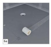
If wedi 610 adhesive sealant has been applied to the building board joints, this is followed by the application of the wedi Tools reinforcement tape.
