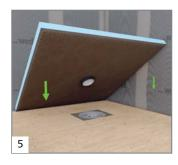
Fit the parts of the drain onto the Fundo element. If necessary, pre-treat the wooden surface with primer before bonding the element. Use tile adhesive to bond the element.
