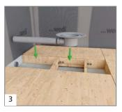
Connection and positioning of the drain body to the pipe. The upper edge of the drain flange should be at the same height as the wooden floor.
