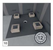
Leave the tile adhesive to settle under low pressure for 12 hours.
