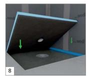
Insert the shower element flush into the recess.
