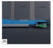
For floor level installation, please be aware of the necessary difference between the top surface of the drain flange and the top surface of the recess.
