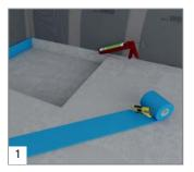
Create a recess in the existing or new screed and attach edge insulating strips if required.
