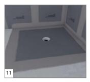
Seal all joints and connection areas as well as transitions by using sealing tape and slurry sealant.
