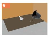
Apply a self levelling screed mix to cover all of the proposed area. This will ensure ShowerDec® is fully supported.
