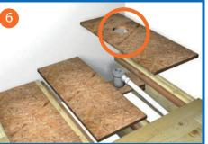
50mm x 25mm runners 18mm down each side of the joists and cross noggin with extra support timbers where necessary. Cut 18mm marine ply panels and insert between the joists and fasten down to the support runners using wood screws.
