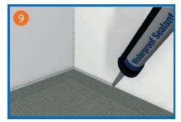
9) Apply a bead of non-solvent based sealant or Jackoboard board fix adhesive to the entire perimeter of the tray and allow to cure.
