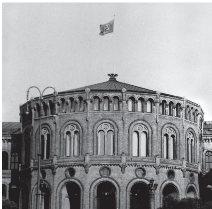
Illustration 4.4: The Nazi flag above the Storting building during WW2. (Gustav Brosing, UBB)
