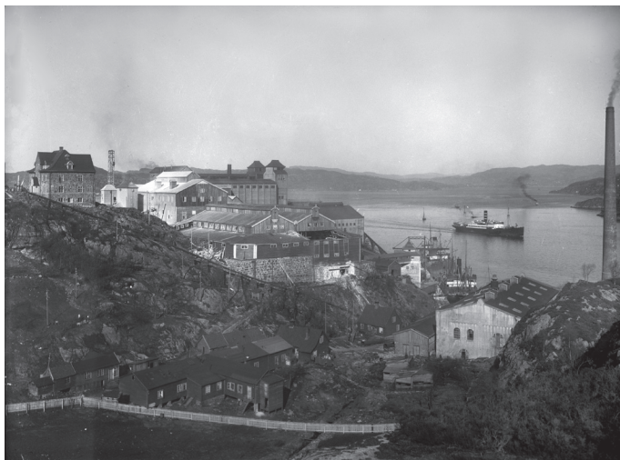
Illustration 4.3: This factory at Knarrevik outside Bergen produced herring oil and fertilizer, and was operated on hydroelectric power. We can see the penstock running down the hill, and the workers' houses beneath. A steam ship is in the fjord. Around 1918. (Atelier KK, UBB)
