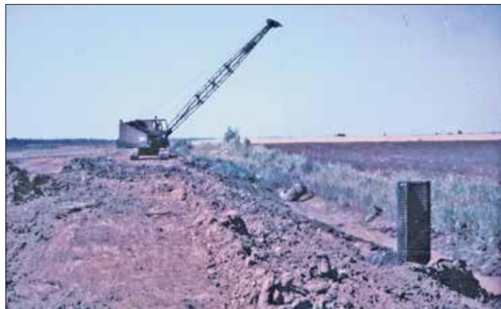
Another view of a field impoundment dike being constructed with the refuge dragline. PHOTOS COURTESY OF TRAVIS H. MCDANIEL
