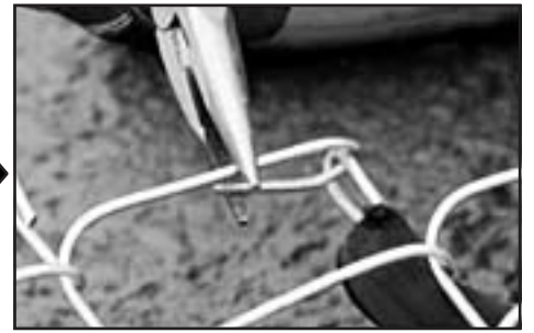
Use pliers to close the Open Knuckle end
