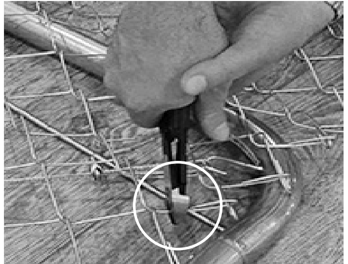
At the bottom of the frame: Cut right before the knuckle loop
