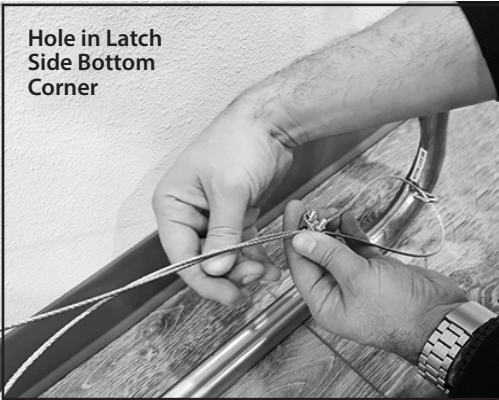
Shown: CORNER HOOKS straight edge connects to pre-drilled hole in corner.
