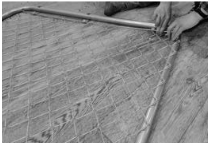
(#1) The remaining mesh section to install the tension rod (C) to (#2) The excess mesh to be discarded
