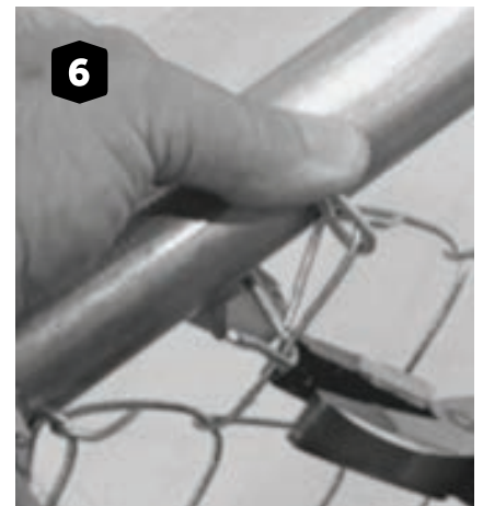
Use pliers to pinch shut the wire tie to secure it to the Closed Knuckle.
