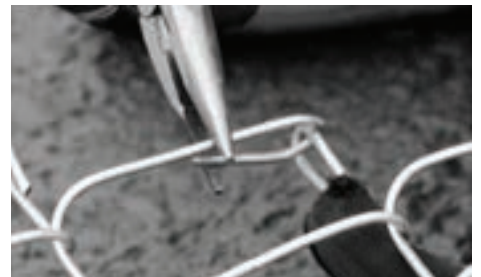
Use pliers to close the open knuckle end.
