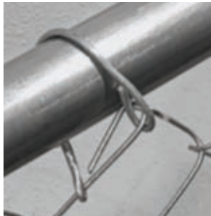
Use pliers to grab the end of the wire tie and wrap it around the same Closed Knuckle you started with.
