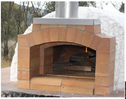
Put a thin bead around the top of the brick exhaust creating a seal and push the stainless cap down to secure ,
