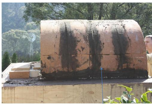
Make sure you have filled in all the gaps in between the joins putting a thin layer of mortar not thicker than 2mm
