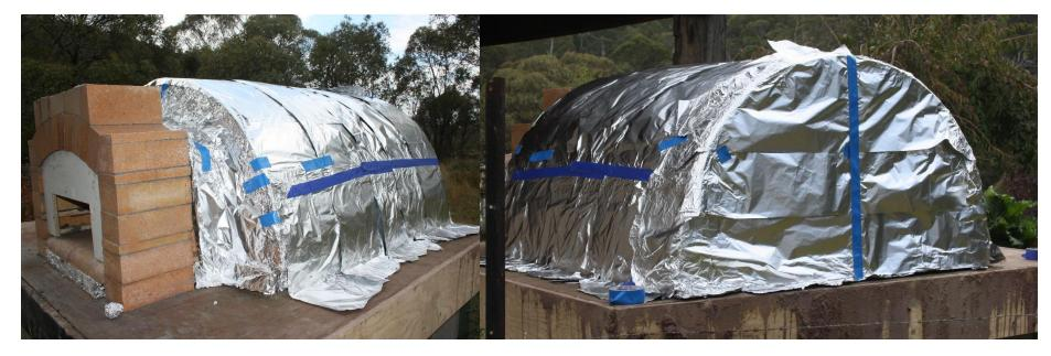
• Before you attempt to insulate the oven wrap the ovens chamber in aluminium foil like a hot potato. You can do 1 layer or 5 layers the more the better. This stops the water from getting into the chamber over time.
