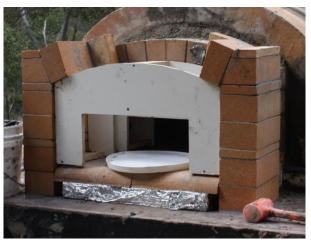
Please start off by DRY laying your front floor tiles including the underfloor tiles then place your template with the spacer/packer under each point of the template. This will be easier to pull the template out at a later stage.
