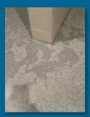
In the early life of the concrete slab, water is present in abundance and must be retained during the initial curing period to produce high quality concrete. However, the concrete must give up most of its water during the subsequent drying period to become suitable for low permeability flooring.
