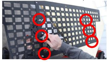
Ensure the top mounting holes in each panel are pointed upward.
