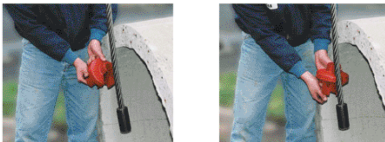
Drop pipe carrier lifting sling through hole in pipe. Align and insert "Tea Cup" pipe carrier into lifting sling.
