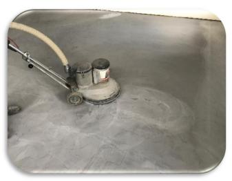
Mix and Apply Primer Coat - Ecoflor® Concrete Modifier. 1 part modifier: 1 part water. Blend the adhesive mix with a purpose made paddle attachment to an appropriate power drill. Once mixed, apply the adhesive to the surface using a broom or roller, ensuring an even coverage of the contents. Allow to dry.
