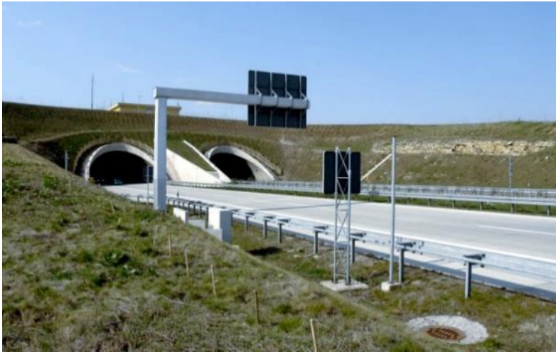
BAB 17 – tunnel Dresden-Coschütz, Germany
