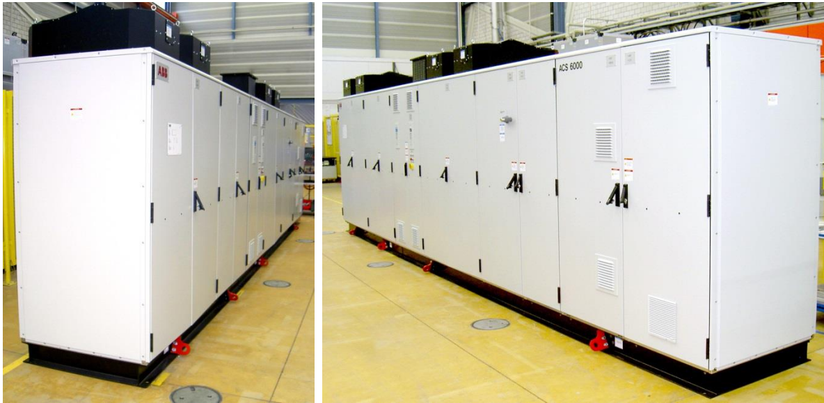
Type: MV converter ACS6000 (ABB) Natural gas storage Staßfurt 5,200 kW, 3,160 V, 597 r.p.m.
