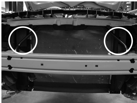
Fig. 5-a: Remove Front Braces
