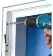
Re hang the panel back onto the male pin on the frame, check closure and alignment and adjust hinges up or down if required.
